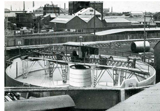
Cement plants that employed the “wet” method of mixing ground limestone and clay typically relied on so-called washmills for the process. This example, from the English operation at Wilmington, was 66 feet across. (Dylan Moore)
