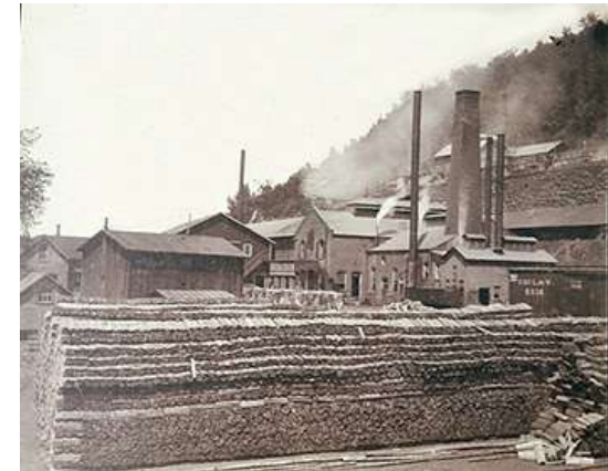
This photographic view of the Consolidated Cement Works at Rosendale reveals first, in the foreground, the enormous stacks of wood needed in the firing of the shaft kiln, the major vertical element seen at right-hand side. Tall metal chimney stacks rise from various areas of the operation. It is presumed that the natural cement mine was situated in the steep hillside. (Werner and Burmeister)
