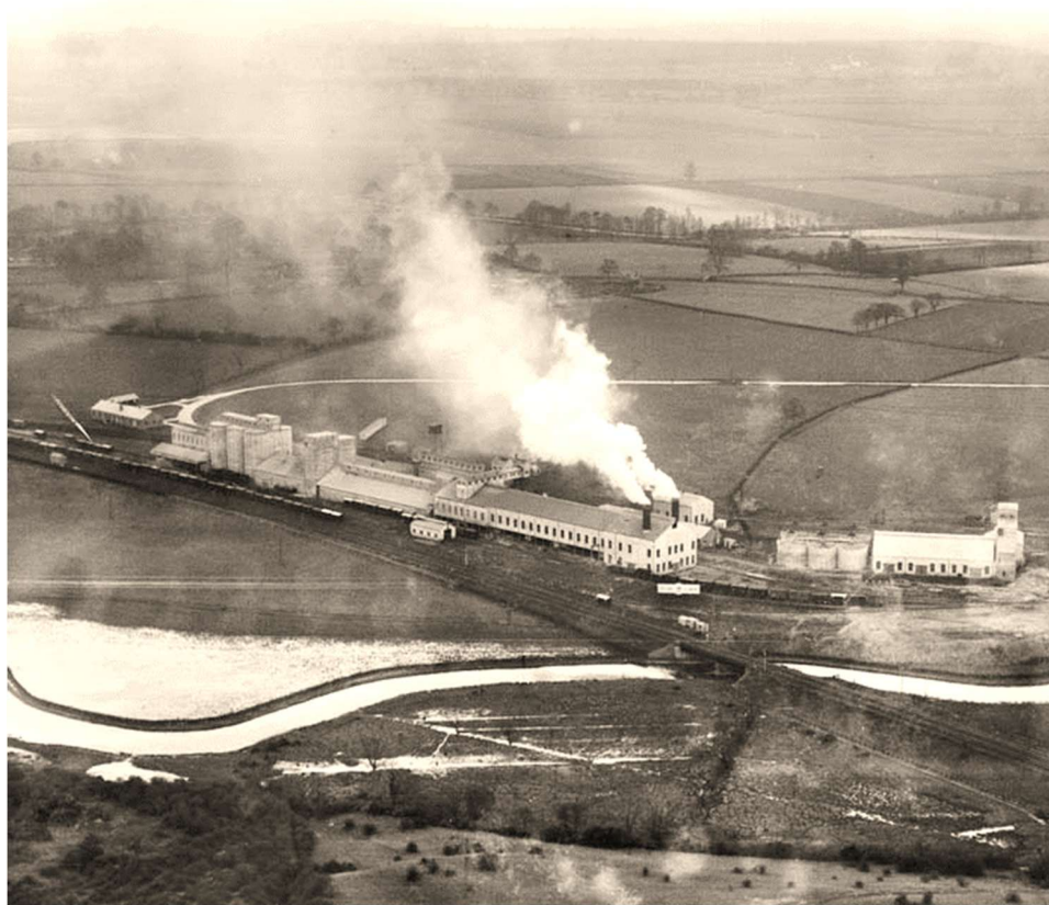
Oxford Cement Plant, in 1930. This operation is more understandable in terms of its layout than many other Portland cement plants, which tend to be more concentrated. Dylan Moore notes: "The plant had a simple linear design, starting with rawmills at the right-hand end, followed by slurry tanks [the large circular forms adjacent], kilns [in the long multi-windowed building, presumably rotary kilns and with twinned stacks exhausting gases, and then the various buildings in a line]: clinker store, finish mills, cement silos and packing and loading plant. The River Cherwell was in the foreground, and the quarry reserve occupied the fields behind the plant." (Dylan Moore)
