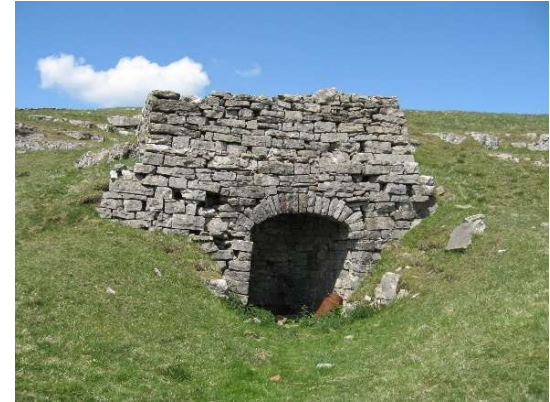
This photograph of an old English pot kiln shows the typical situation for such operations – set into a hillside, to allow easier access at both key levels of the structure – at the top, where limestone chunks and wood or coal would be deposited, and at the bottom where the residue would be removed. This or smaller versions like this would have been found in many areas of Manitoba. (Wikimedia Commons)
