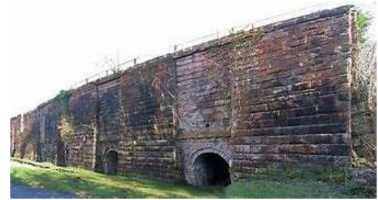
Froghall Lime Kilns, in Staffordshire, England. (Froghall Historic Site)
