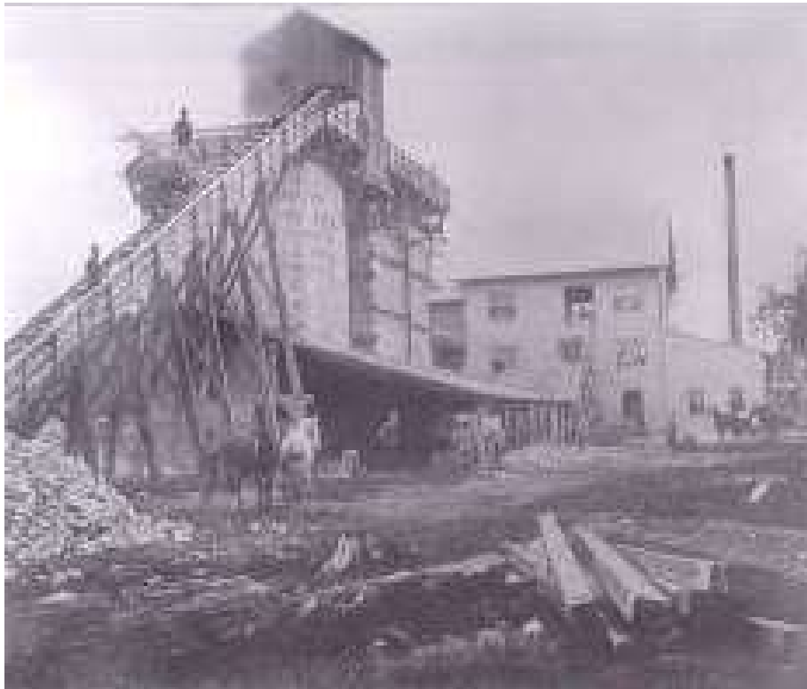
This image is thought to show one of the Rosendale natural cement operations. (Wikimedia Commons) Note the two stout stone kilns and the steeply-angled ramp used to move raw material via carts into position. Also note the housing atop the kilns, presumably where workers would tip the carts and then pour contents into each kiln mouth. A shed-roofed passage at the base of the kilns led to the three-storey processing site – presumably for final grinding and bagging. The tall stack in the right-hand distance would have been used to exhaust the various pieces of machinery inside.
