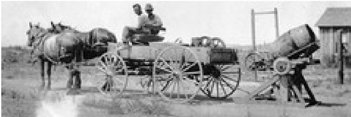
An early image of a cement mixer, attached to the back of a wagon.
