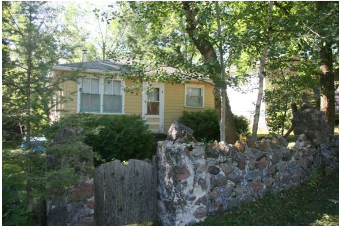
View of the “Summerhill” Cottage, showing a range of stone features.
