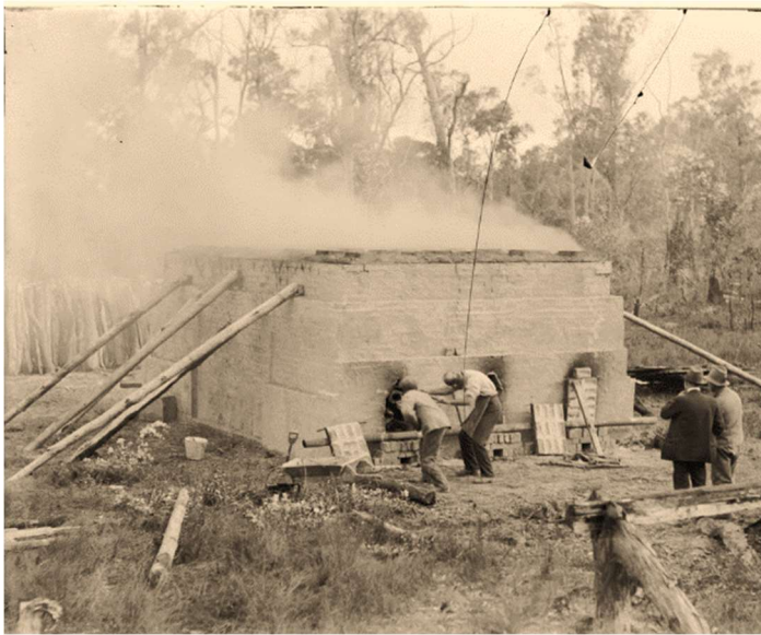
Archival view of an English scove kiln in operation, ca. 1900. The scove kiln was a permanent structure loaded with green bricks and then fired via small doors at the base. This type of kiln produced much better results compared with the clamp kiln. In both cases several thousands of brick could be burned at a time, over several weeks of operation for a single “burn.”
