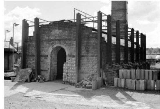
Example of a tunnel kiln at the Ochiltree-Burnfoot Tile Works in Scotland. The distinctive barrel vault and metal support structure are visible here. The large arched door would have been bricked in when a burn was underway. (Scottish Brick History)
