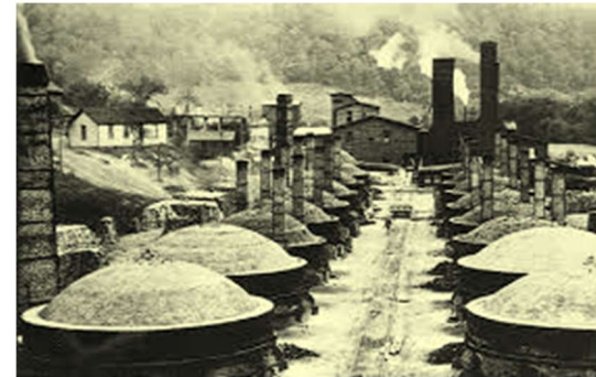
A view of multiple beehive kilns and chimneys at the brick factory at Clay City, Washington, 1910. Combining a number of beehive kilns and chimneys was a common way to develop an especially large clay or shale deposit at this period of the North American brick-making industry.
