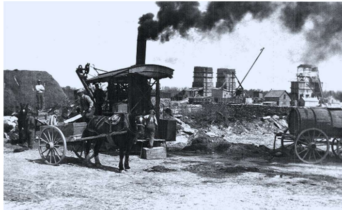
Left, top: A steam excavator was used to clear the overburden from the limestone rock (Stonewall. Turning a Century. 1878-1978).
