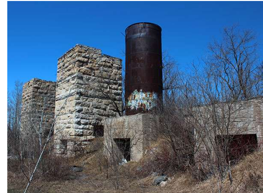
In recent years, lime was produced at the Gillis Quarry at Garson in two large stone shaft kilns and two smaller pot kilns, with steel tube chimneys (Manitoba Historical Society).
