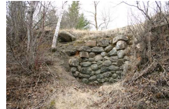
Contemporary view of the Birtle Lime Kiln, showing the face of the kiln, built up with granite fieldstones, which would have sheltered a depression behind it and set into the hillock. The granite stones presumably could withstand the heat of the fires consuming the limestone chunks in the kiln.
