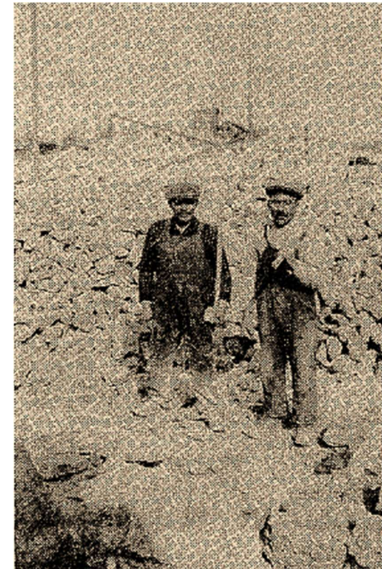
Fred Klimchuk and Sam Kisiow breaking limestone by hand for burning in a lime kiln (From They Stopped at a Good Place ).
