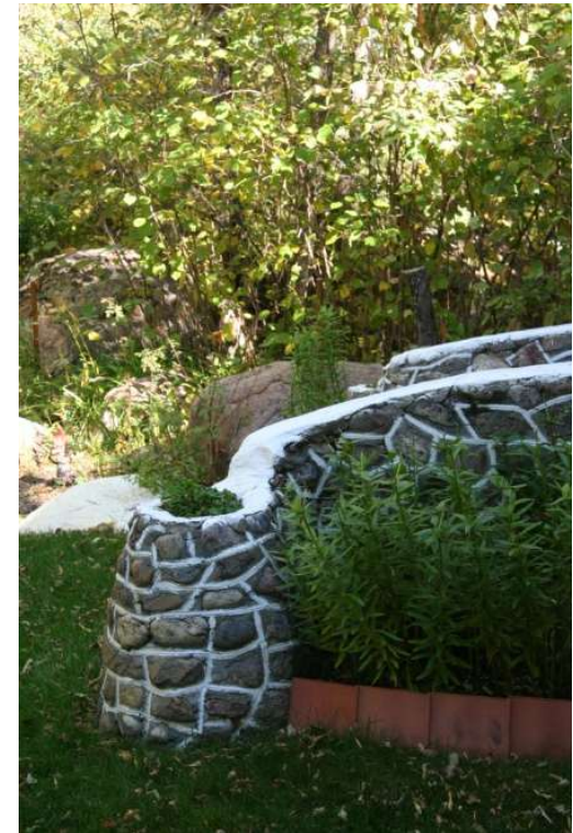
An exceptional example of the “Grand Marais” stair, here with stones finely picked out with white-painted mortar – very elegant.
