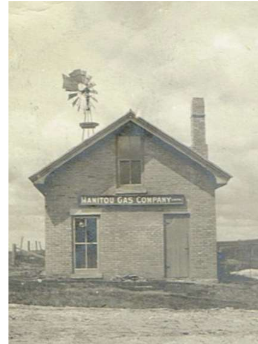
View looking to the west of the Manitou Gas Company plant, ca. 1915.
