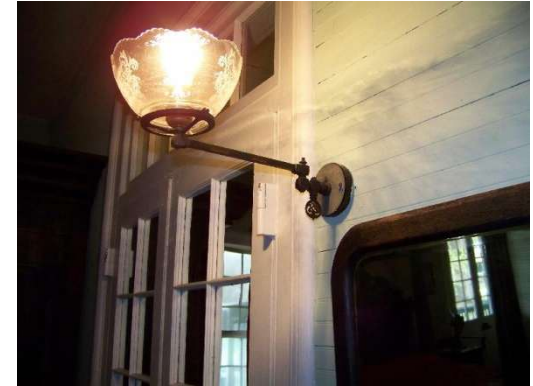
Example of a domestic gas lamp, showing the lamp and armature that provided gas to the light.
