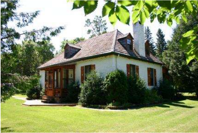
East Selkirk Area, Bunn Road GPS Reading: N 50° 8.435 W 96° 50.520
